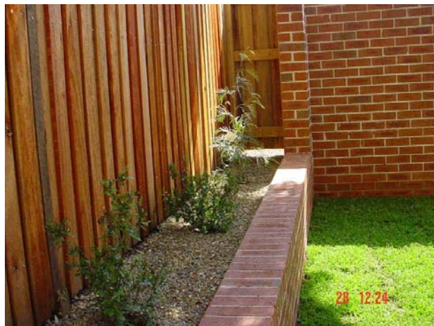
A photo of a minor overland flow path.
