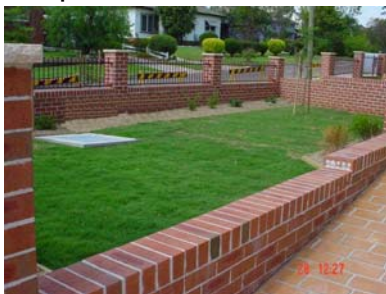
Typical Above Ground OSD System (Most Common).
